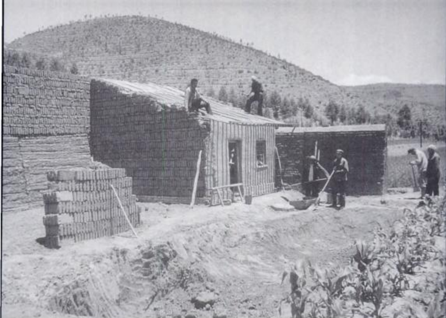
65. Farmers are building a barn next to their homestead. Their primary building material is adobe blocks. Photo: Zhou Pengqi
